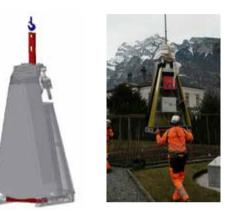
Remove forklift protection before fixing on the foundation is done otherwise when already fixed to the foundation resulting tension will not allow to remove the forklift protection any more!
