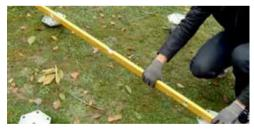
Maximum distance between foundation and frame 2 mm otherwise install steel shims between
