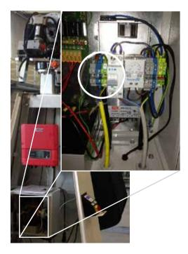
• Installation of anemometer is done by connecting the anemometer-plug to the control cabinet. If it is necessary to remove the plug (i.e. due to cable mounting) it is possible to unscrew the plug, remove it and attach it again after the cable is laid properly. The pins at the plug as well as each cable end are numbered from 1 to 4.
